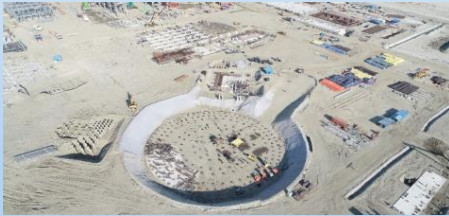
Piling works of Boiler Chimney
