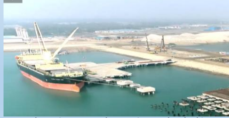
Vessel carrying Power Plant Equipment berthed in unloading Jetty of newly constructed port
