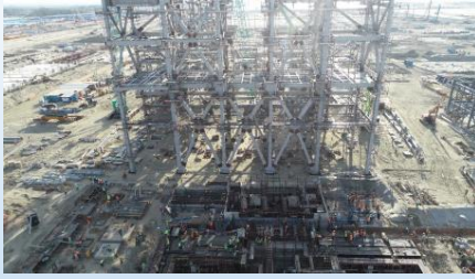
Steel Structure Erection works of Boiler
