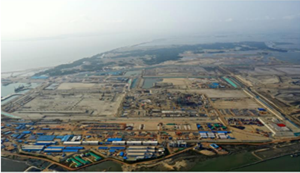
Overall Construction Progress of Power Plant Area till May 2021
