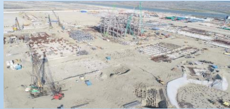
Piling & Civil Foundation works in Power Plant Area
