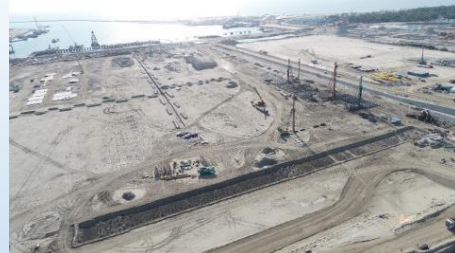
Piling works of Coal yard Area
