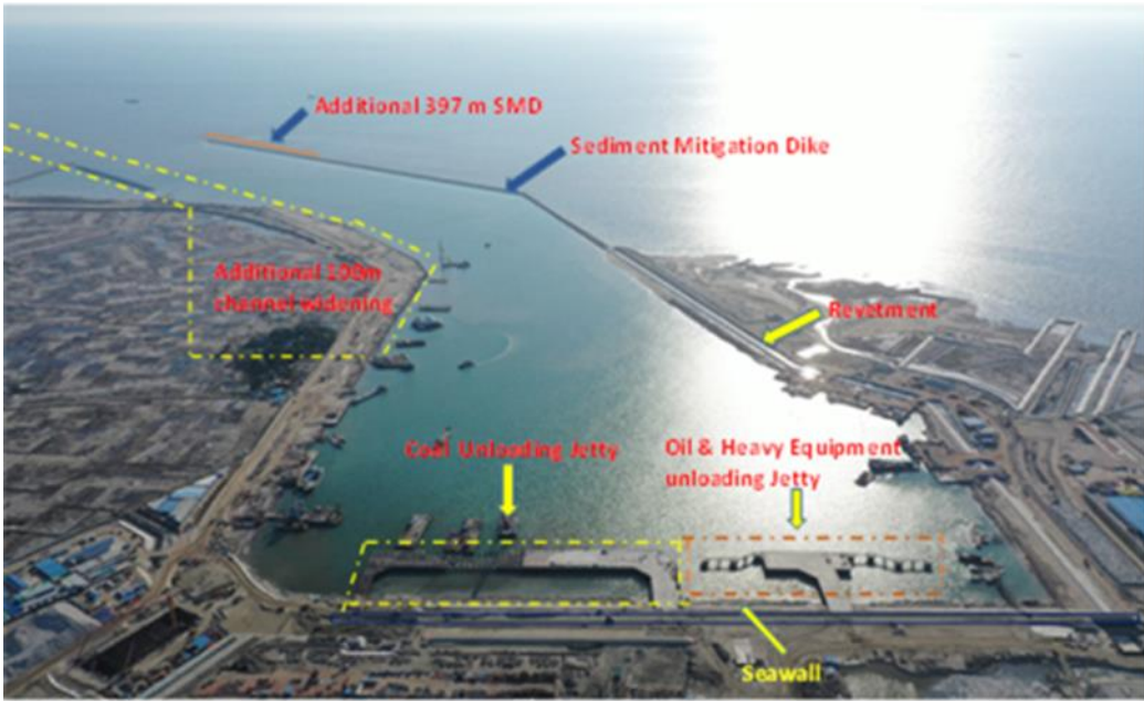
Port Construction Progress till May 2021
