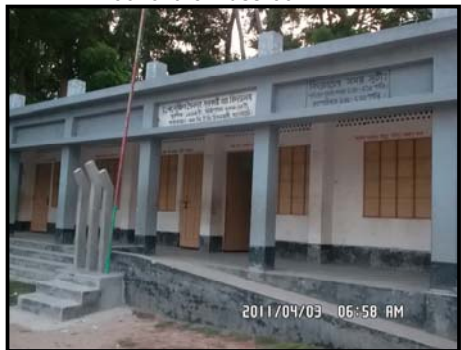
Ramp of the school
