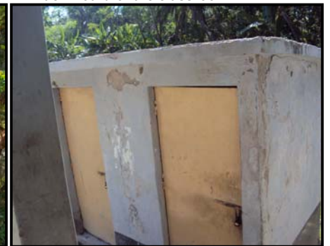
Toilet of the school
