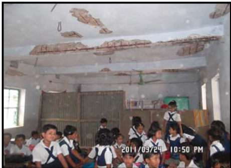
Roof of the Classroom
