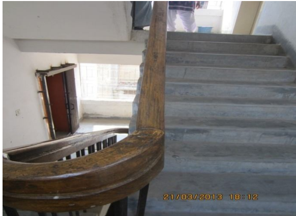
Plate-53: Railing of the building NHB-1/1 showing good condition
