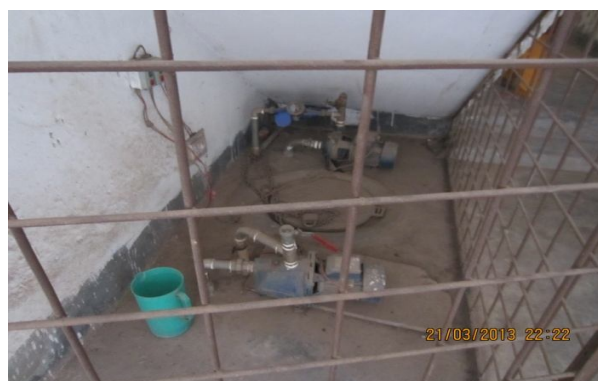
Plate-80: Water reservoir and pump of the building NHB-15/4 under 800 sft flat category
