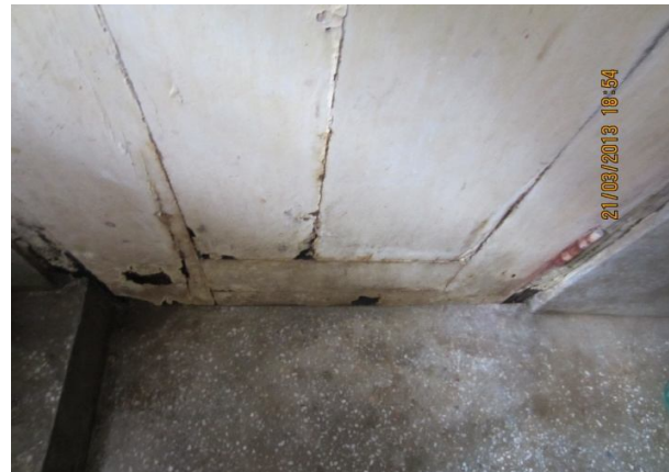
Plate-70: Damaged wooden door of bathroom in the flat B-1 of building NHB-3/2 of 800 sft flat
