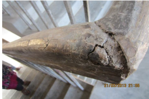
Plate-54: Railing of building NHB-5/1 showing damaged condition under 800 sft flat type
