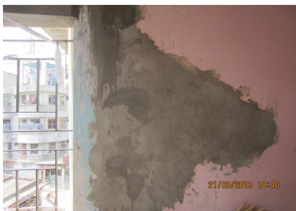
Plate-65: Repaired plaster of wall of dining room in the flat A-2 of building NHB-3/1 of 800 sft flat
