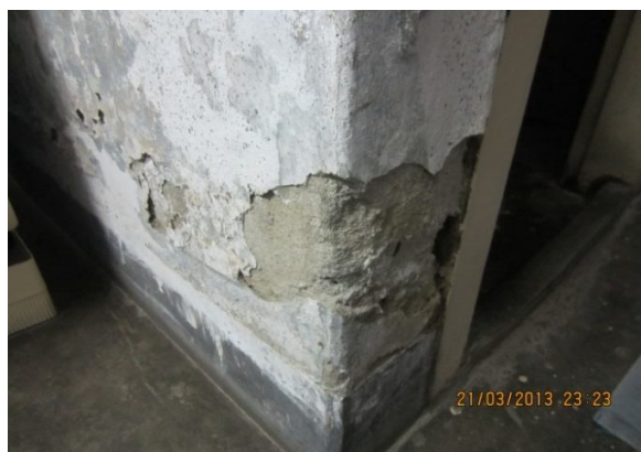
Plate-64: Damaged wall of dining room in the flat A-4 of building NHB-13/3 of 500 sft flat type
