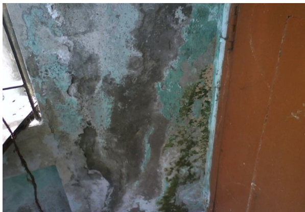
Plate-25: Damaged plaster of the bed room wall in the flat A-3 of NHB-11 under 1000 sft flat category
