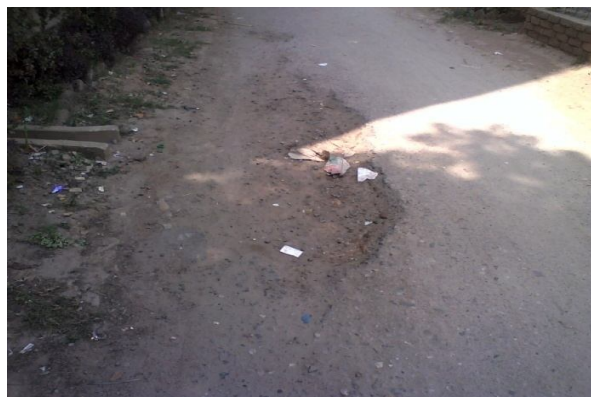
Plate-4: Damaged pavement on the road at the eastern side of the building no. 11 in 1000 sft flat area
