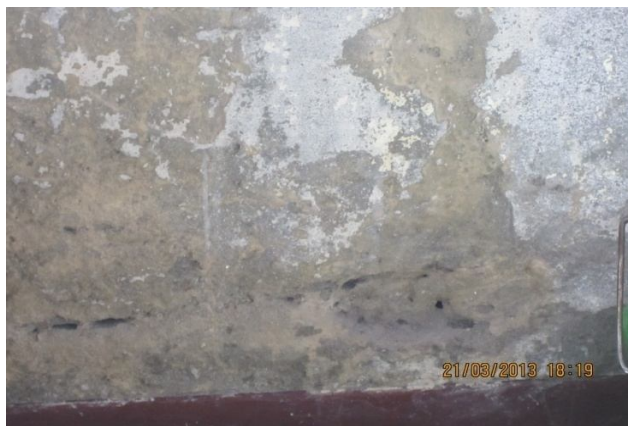
Plate-55: Damage plaster of bed room wall in the flat B-2 of building no. NHB-1/1 of 800 sft flat
