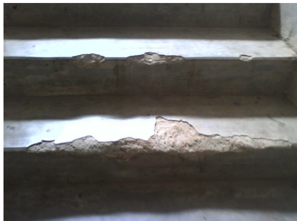
Plate-10: Plaster of stairs of building NHB-4 showing damaged condition
