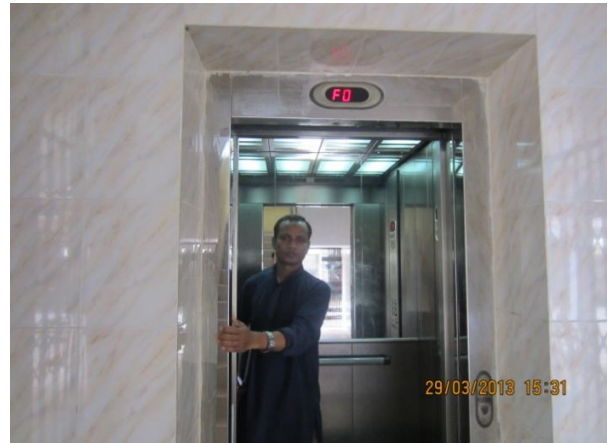
Plate-9: Remodeled and improved condition of outer construction structure of lift in building NHB-1
