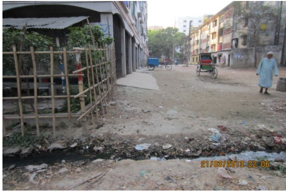
Plate-41: Damaged pavement on the road in front of the building NHB-5/2 of 800 sft flat area
