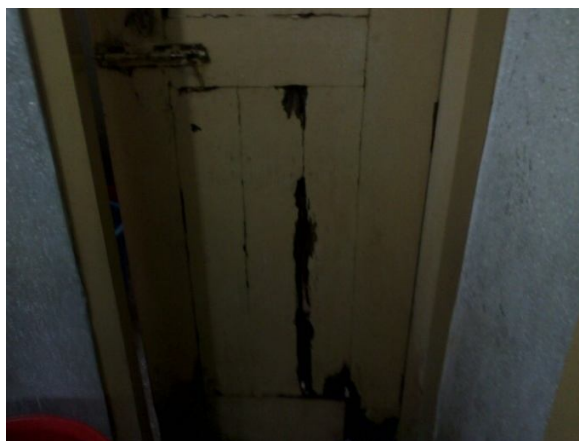
Plate-28: Severely damaged wooden door of the bath room in the flat A-2 of building NHB-4
