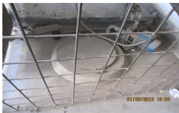
Plate-79: Water reservoir and pump of the building NHB-1/1 under 800 sft flat category
