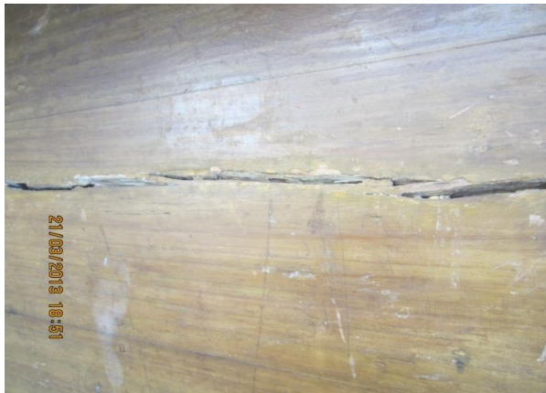
Plate-69: Cracked wooden door in the flat B-1 of building NHB-3/2 of 800 sft flat type
