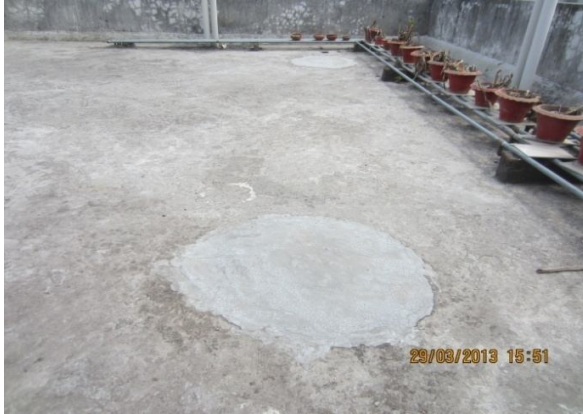
Plate-16: Repaired potholes on the roof of the building NHB-1 under 1000 sft flat category
