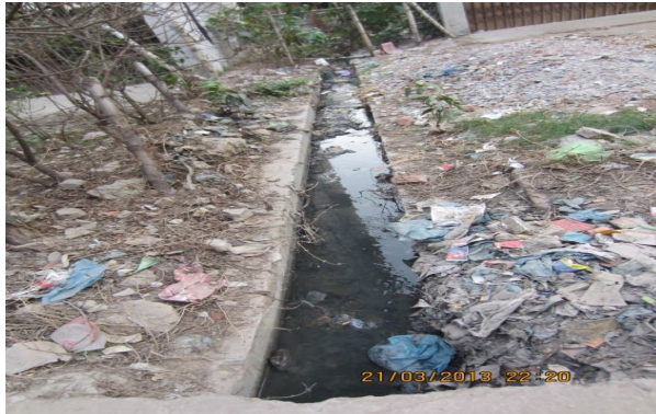
Plate-47: Drain near the building NHB-10/B-2 of 800 sft flat category found in filled with garbage
