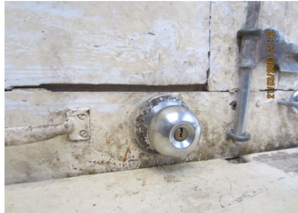
Plate-74: Cracked door in the flat A-1 of building NHB-5/1 under 800 sft flat category
