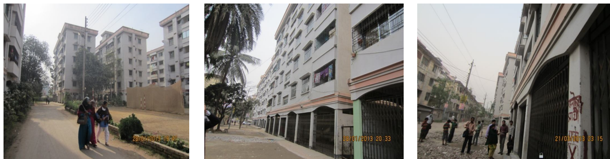
Plate-3: External view of buildings having 800 sft (left), 800 sft (middle) and 800 sft (right) flats located in Mirpur-2 and Mirpur-14, Dhaka
