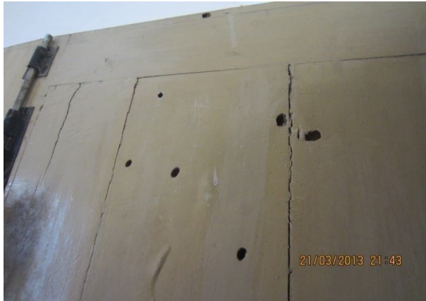
Plate-73: Damaged wooden door of bed room in the flat B-1 of building NHB-5/1 of 800 sft flat
