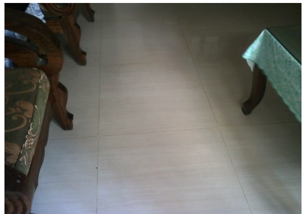
Plate-24: Modified floor by replacing with tiles in the flat B-2 of NHB-6 under 1000 sft flat category
