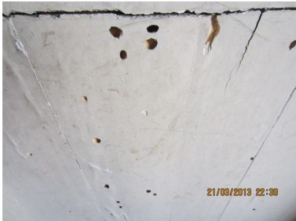
Plate-75: Damaged wall of bed room in the flat A-3 of building NHB-15/4 of 500 sft flat category
