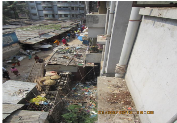
Plate-44: Drain behind the building NHB-3/2 found in filled with garbage in 800 sft flat area
