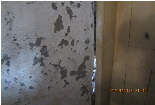
Plate-59: Damaged wall of bed room in the flat A-1 of building no. NHB-5/1 of 800 sft flat
