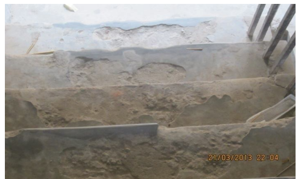
Plate-50: Plaster of stairs of the building NHB-5/1 showing severely damaged condition
