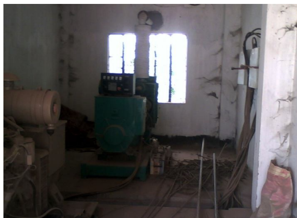
Plate-36: Generator for emergency power supply in the flats under 1000 sft flat category
