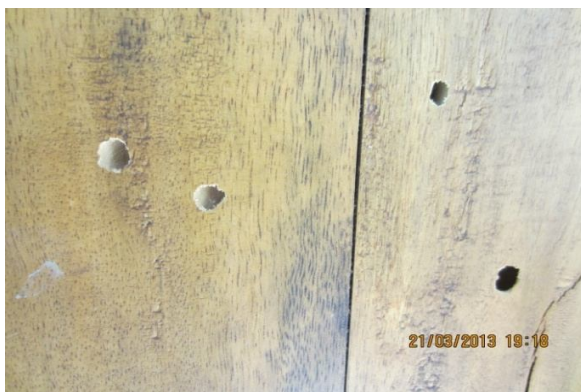
Plate-71: Damaged wooden door of bed room in the flat A-1 of building NHB-3/3 of 800 sft flat
