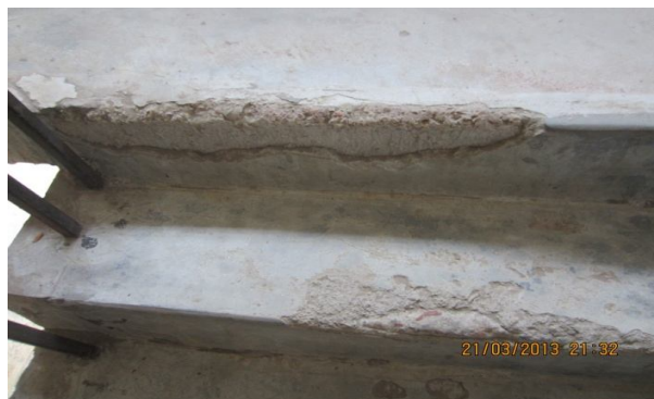
Plate-49: Plaster of stairs of the building NHB-5/2 showing damaged condition
