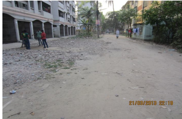
Plate-42: Damaged pavement on the road in front of the building NHB-10/2 of 800 sft flat area
