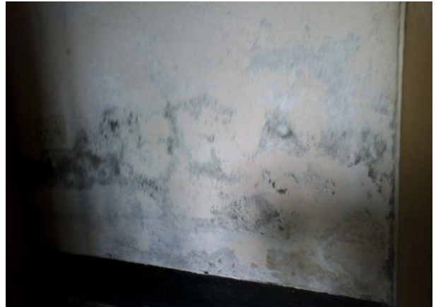
Plate-22: Damaged plaster of bed room wall in the flat B-2 of NHB-4 under 1000 sft flat category
