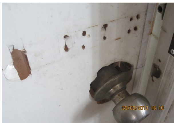
Plate-29: Severely damaged plastic door of the bath room in the flat A-4 of NHB-1
