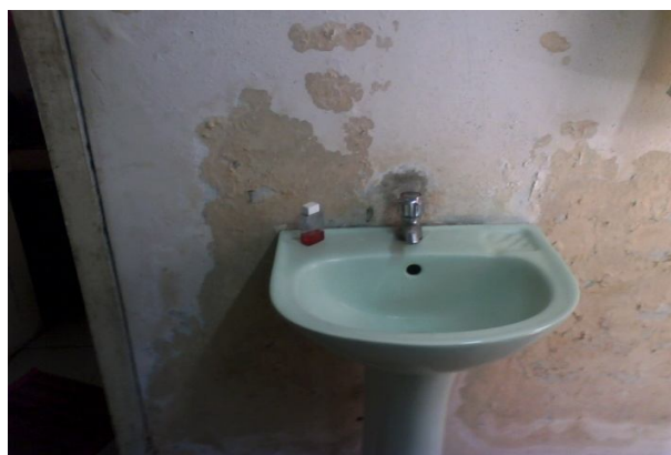
Plate-32: Damaged wall of bath room in the flat B-2 of NHB-6 under 1000 sft flat category
