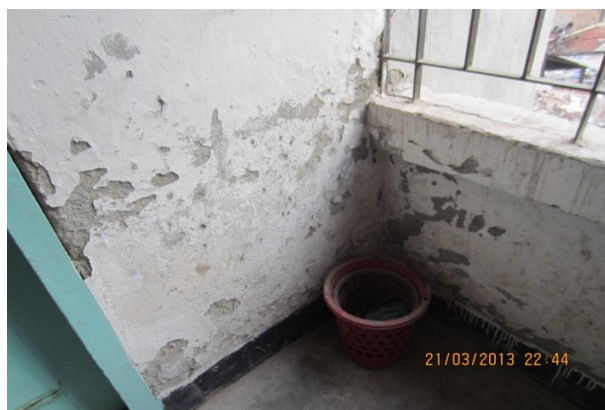
Plate-63: Damaged wall of bed room in the flat A-1 of building NHB-15/5 of 500 sft flat type
