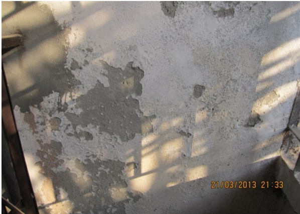
Plate-57: Damaged plaster of bathroom in the flat A-2 of building NHB-5/2 of 800 sft flat
