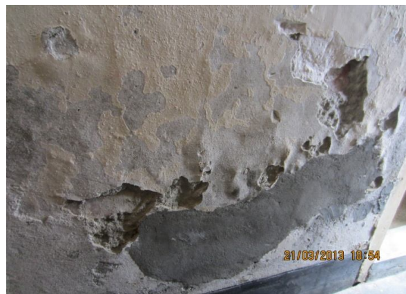
Plate-56: Damaged wall of bathroom in the flat B-1 of building NHB-3/2 of 800 sft flat
