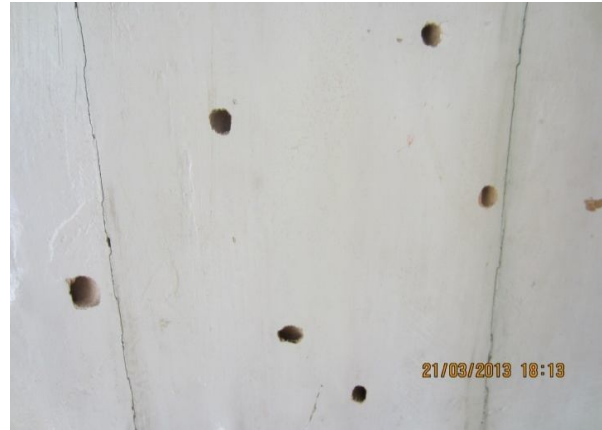
Plate-68: Damaged wooden main door showing holes caused by wood boring beetle (insect) in the flat B-3 of building NHB-1/1 of 800 sft flat type
