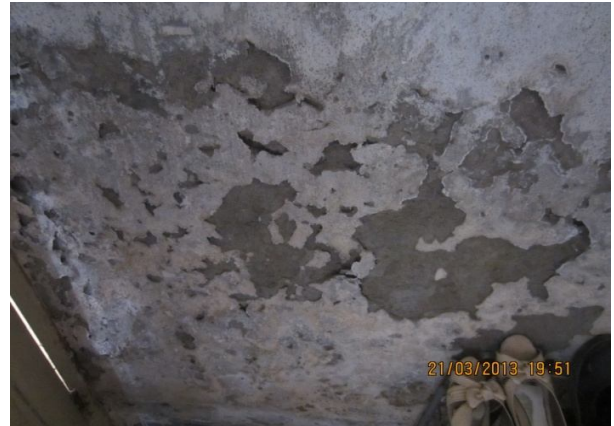
Plate-58: Damaged plaster of bathroom wall in the flat B-2 of building NHB-6/2 of 800 sft flat
