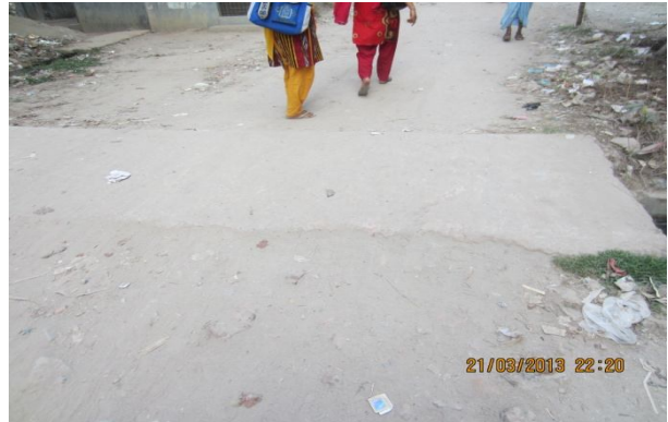
Plate-48: Culvert on the road in the 800 sft flat area
