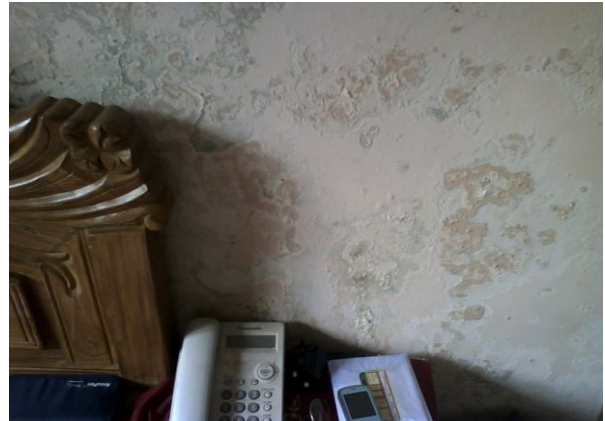
Plate-20: Damaged plaster of bed room wall in the flat B-1 of NHB-3 under 1000 sft flat category
