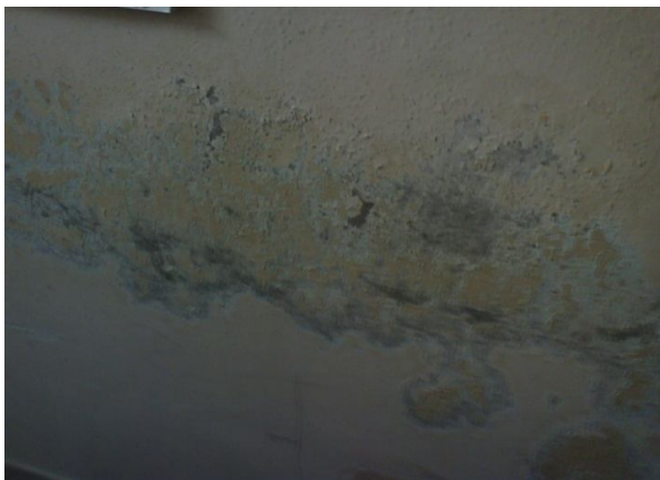
Plate-23: Damaged plaster of bed room wall in the flat B-2 of NHB-6 under 1000 sft flat category
