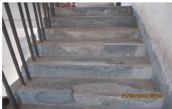
Plate-51: Plaster of stairs of the building NHB-6/2 showing damaged condition
