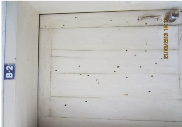
Plate-67: Severely damaged main door showing holes caused by wood boring beetle (insect) in the flat B-2 of building NHB-1/1 of 800 sft flat
