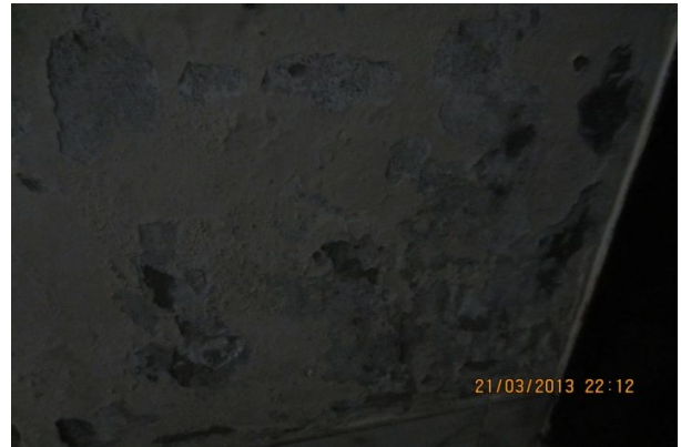
Plate-60: Damaged wall of bathroom in the flat B-1 of building NHB-10/B-2 of 800 sft flat
