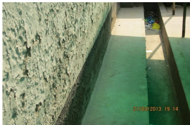
Plate-46: Wall base near the drain of building no. NHB-3/2 found in damp and damaged condition in 800 sft flat area
