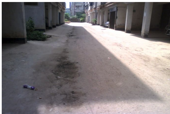
Plate-5: Damaged pavement on the road in front of the building no. 13 in 1000 sft flat area
