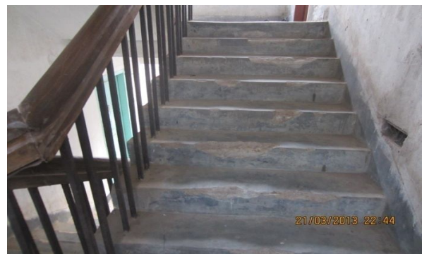
Plate-52: Plaster of stairs of the building NHB-15/5 showing damaged condition
