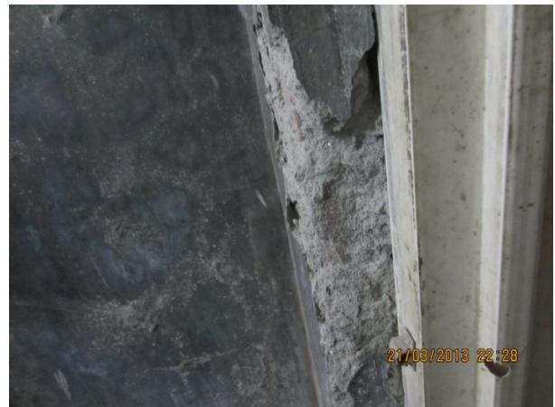
Plate-62: Damaged wall of bathroom in the flat A-1 of building no. NHB-15/4 of 500 sft flat type
