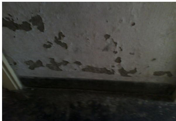
Plate-26: Damaged wall of bed room in the flat A-4 of NHB-16 under 1000 sft flat category
