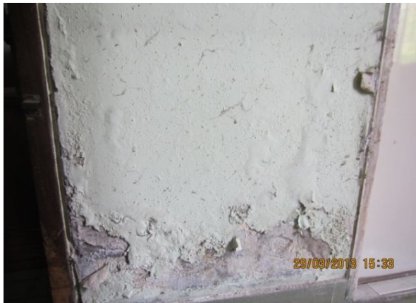
Plate-17: Damage plaster of bathroom wall in the flat B-1 of NHB-1 under 1000 sft flat category
