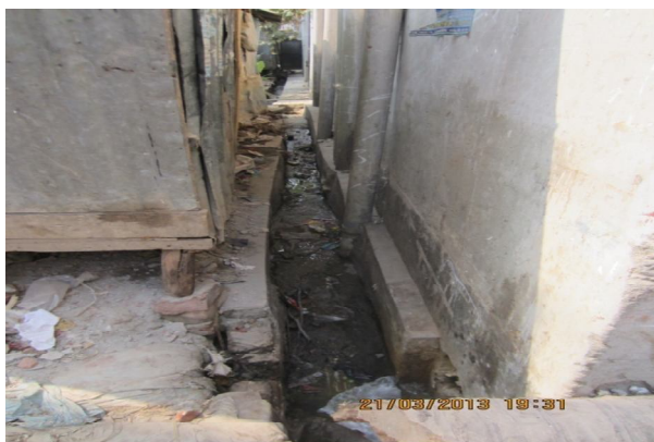
Plate-45: Drain behind the building NHB-3/4 found in filled with garbage in 800 sft flat area
