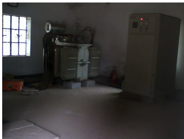
Plate-35: Sub-station for power supply in 1000 sft flat area
