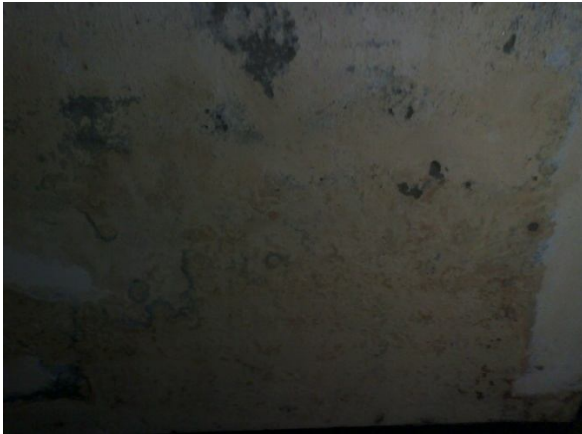
Plate-21: Damaged plaster of bed room wall in the flat B-1 of NHB-5 under 1000 sft flat category
