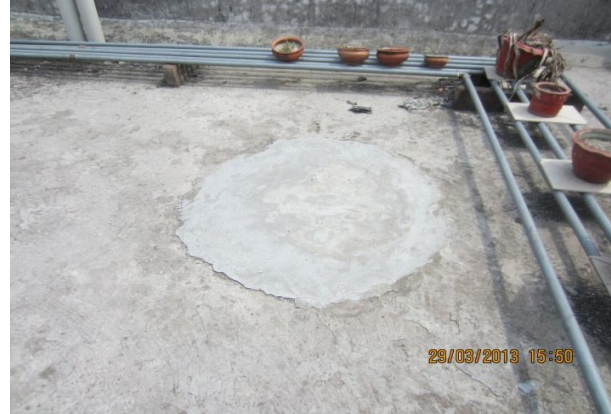
Plate-16: Repaired potholes on the roof of the building NHB-1 under 1000 sft flat category
