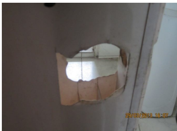
Plate-30: Severely damaged plastic door of the bath room in the flat B-4 of NHB-1
