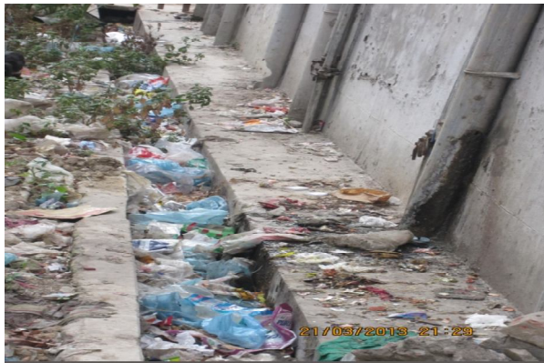
Plate-43: Drain behind the building NHB-6/2 found in filled with garbage in 800 sft flat area
