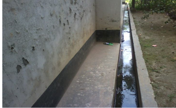
Plate-7: Wall base near drain of NHB-9 found in damp and damaged condition in 1000 sft flat area
