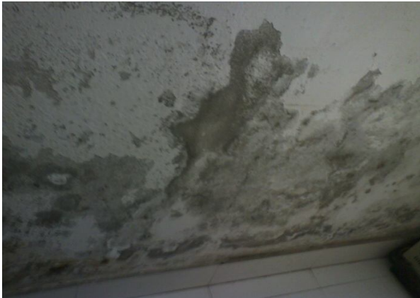
Plate-19: Damaged wall of dining room in the flat A-1 of NHB-2 under 1000 sft flat category
