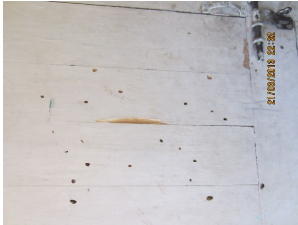
Plate-76: Damaged wooden door of bed room in the flat B-3 of building NHB-15/4 of 500 sft flat
