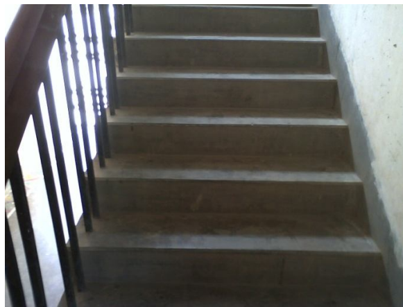
Plate-11: Stairs of building NHB-16 showing good condition
