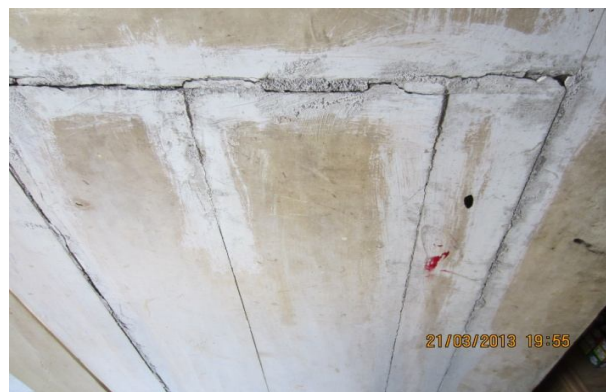
Plate-72: Damaged wooden door of bed room in the flat B-2 of building NHB-6/2 of 800 sft flat
