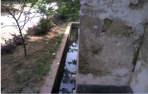
Plate-6: Wall base near drain of NHB-7 found in damp and damaged condition in 1000 sft flat area
