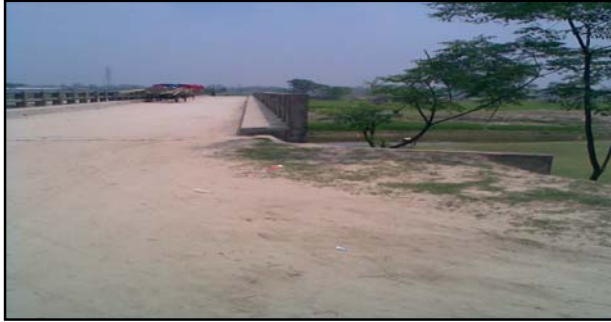
Bbridge on Saidpur-Dinajpur to Botlagari-Paraghat Road over Khorkhoria River, Upazila: Saidpur, District : Nilphamari
