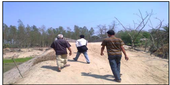
Bridge on Shildabari-Baithabhanga Road Over WAPDA Khal, Upazila: Gabtolia, District: Bogra
