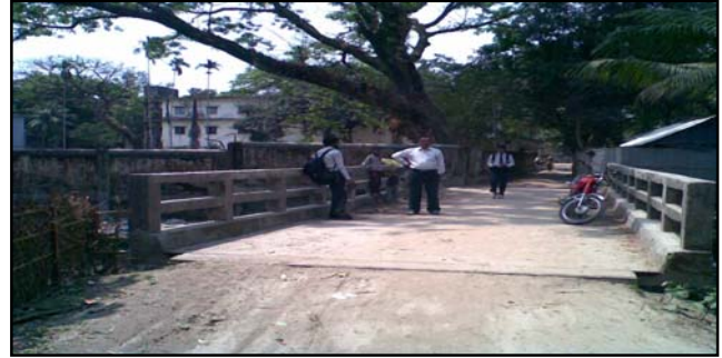
Bridge on PTI Masterpara –Bamandanga Road over Bamandanga River, Upazila: Sadar, District: Nilphamari,
