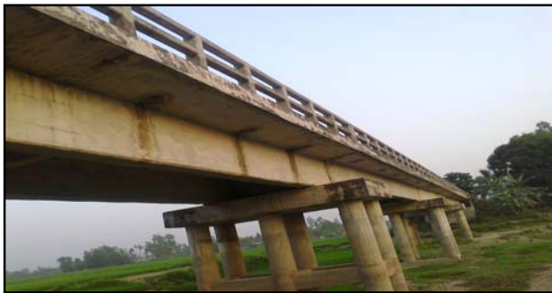
Bridge over Jorhdighi khal, Upazila: Dhunot, District: Bogra
