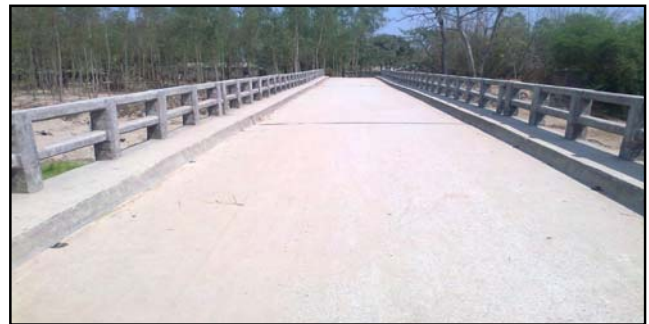
Bridge on Mirzapur-Shughat Road over Bangali River, Upazila: Sherpur, District: Bogra
