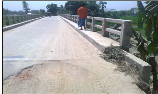
Bridge on Jorhdighi khal, of Dhunot Upazila, under Bogra District
