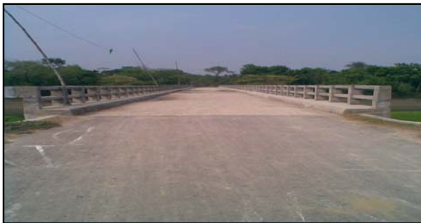
Bridge on Bajitpur-Salainagar Road over Boral River, Upazila: Bghatipara, District: Natore
