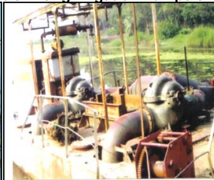
25 cusec double lifting pump
