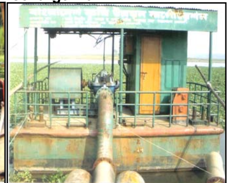
12.5 cusec double lifting pump
