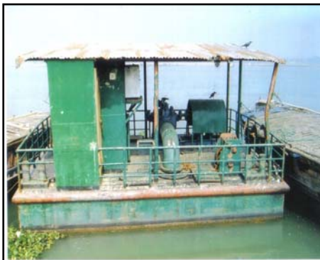
12.5 cusec double lifting pump
