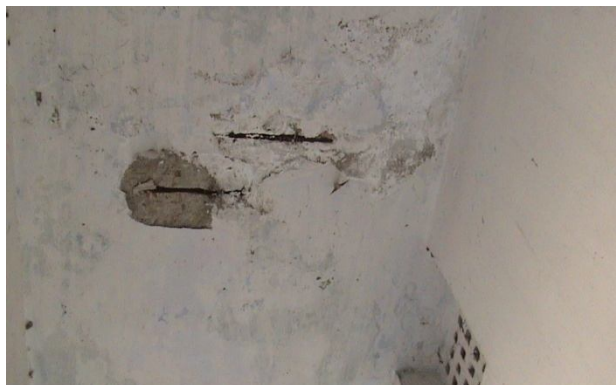
Plate 3.3: Partly removed wall plaster of Kazipur godown, Sirajganj
