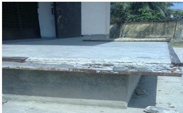
Plate 3.4: Cracked and broken corridor of Kazipur godown
