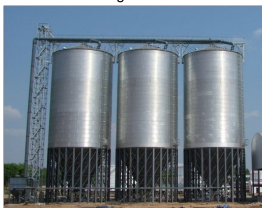
Plate-5.3: Hopper Bottom Steel Silo
