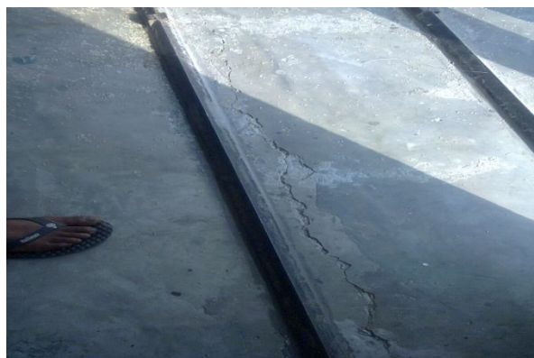
Plate 3.6: Sporadic cracked floor of the Belkuchi food godown, Sirajganj
