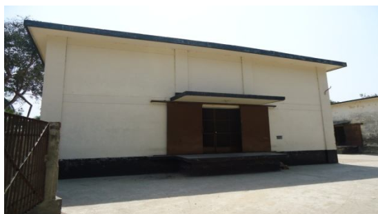
Plate-3.1: New food godown at Thakurgaon
