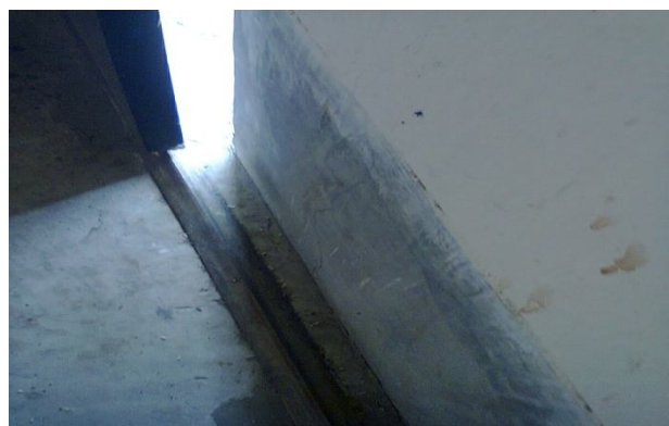
Plate 3.5: Deformed door unable to lock at Kazipur godown, Sirajganj
