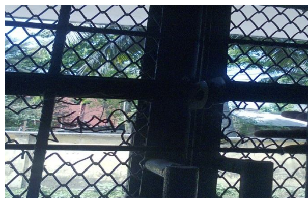
Plate 3.8: Broken main steel door of Natore Sadar food godown
