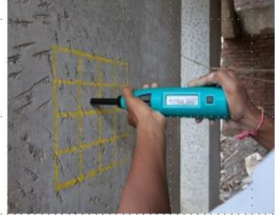
Hammer / Rebound Test
