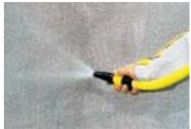
Fig: Curing to be ensured for 28 days
