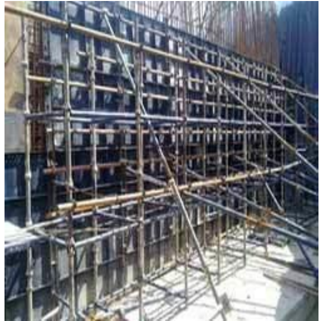
Fig: Shuttering arrangements
