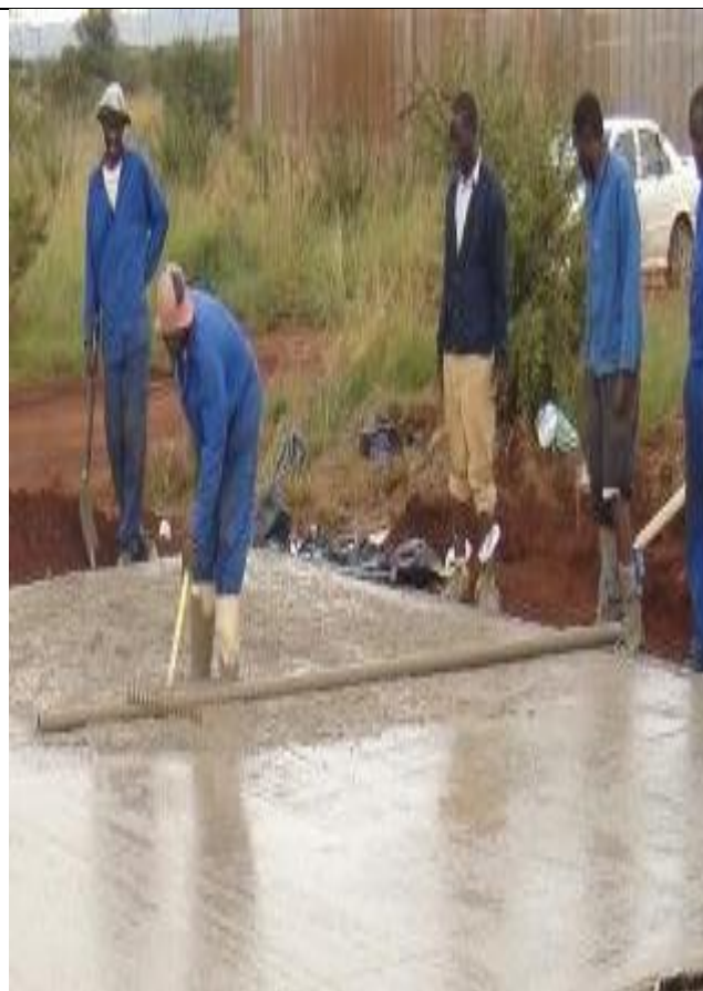
Fig: Foundation casting
