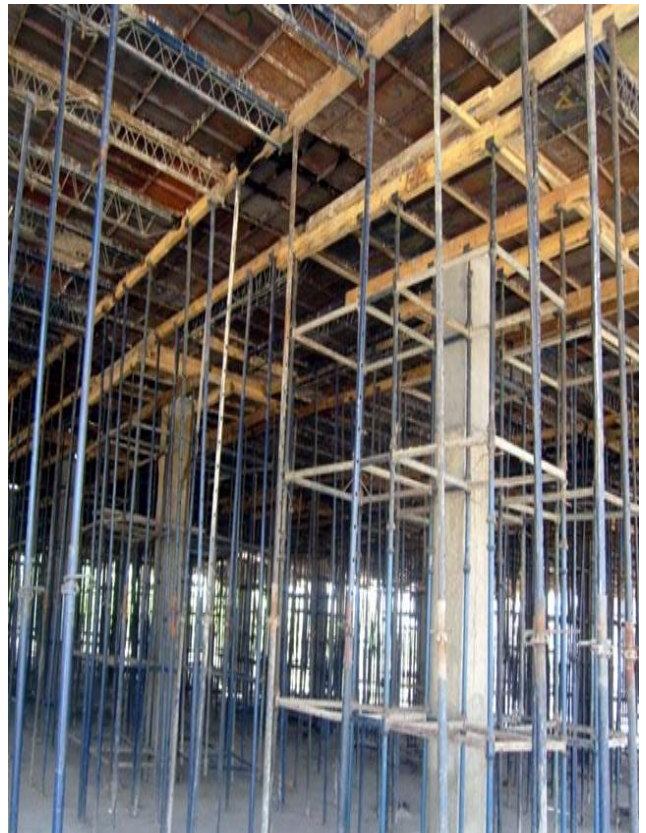
Fig : Use of steel as shuttering materials
