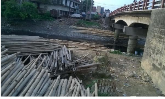
Rajakhali bridge_2-Left side
