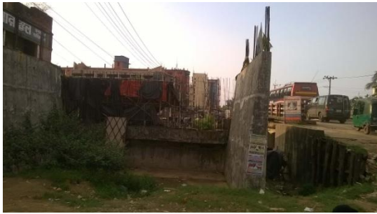
Rajakhali bridge_1-Left side
