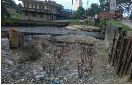
Hafe bazar bridge-Left side
