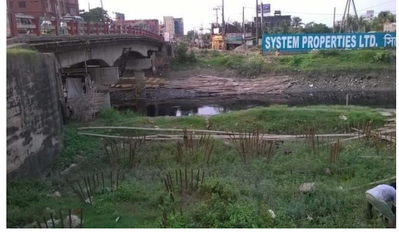
Rajakhali bridge_2-Right side
