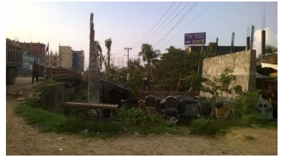
Rajakhali bridge_1-Right side
